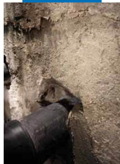
Uzavretie Mapeproof Swell cementovou maltou Mapegrout T40
